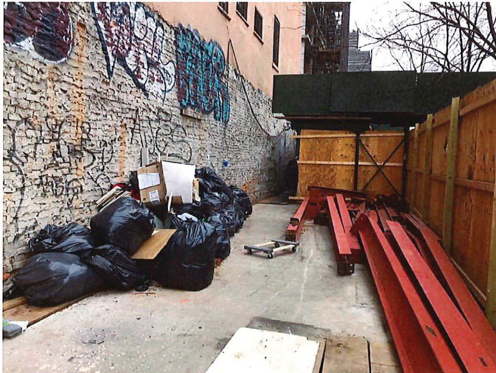
Second Floor Terrace (Structure not yet complete)
